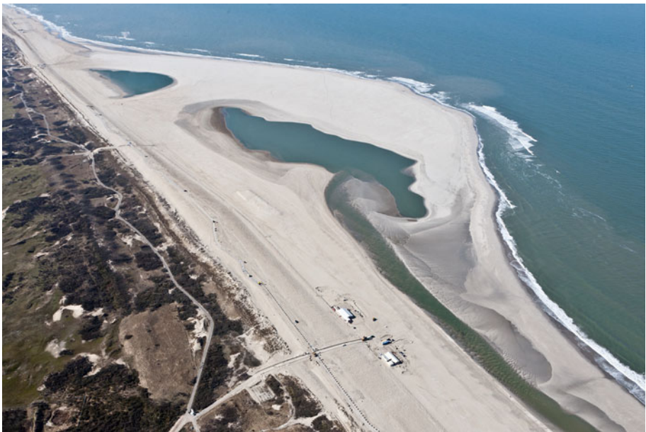
Fig. 7 Aerial view of the Delfland Sand Engine from the northeast, March 2012 (photograph: Rijkswaterstaat/Joop van Houdt)
